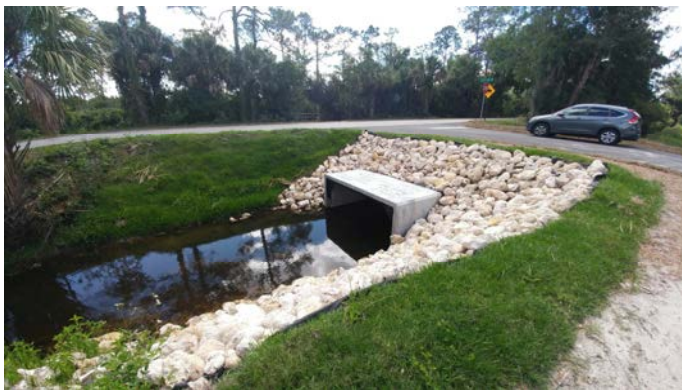
Figure 14. Canal Culvert under 175th
