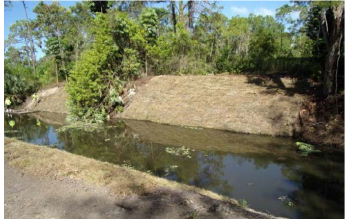
Figure 13. Completed Slope Repair
